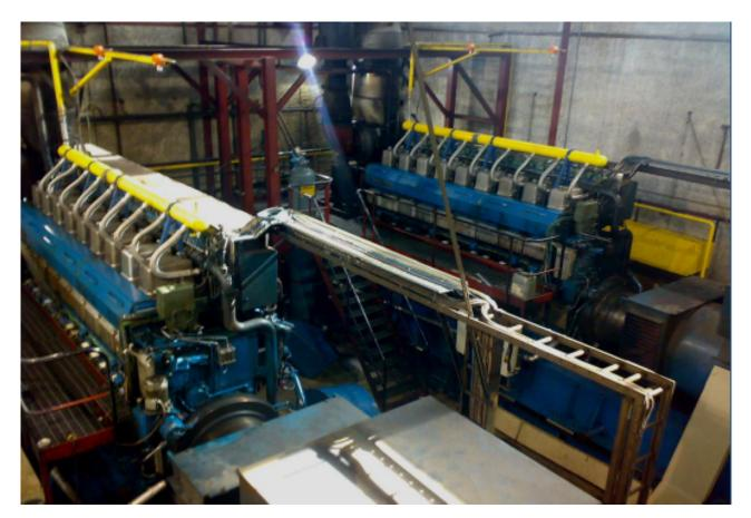
VTec Technology was used to convert two 4.0MW Diesel Engines to Natural Gas but can be used for H2 at Estarreja Portugal.
